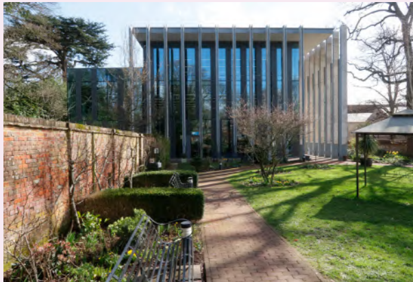
Bourne Hill Council Offices, Salisbury
