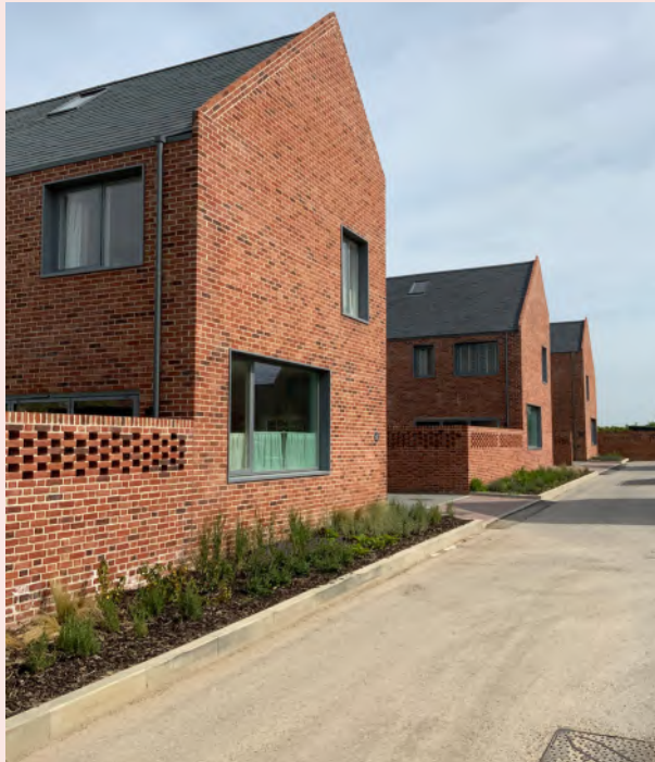
Side gables include large windows to habitable rooms. Boundary walls include perforated brickwork. The Tannery, Holt.
