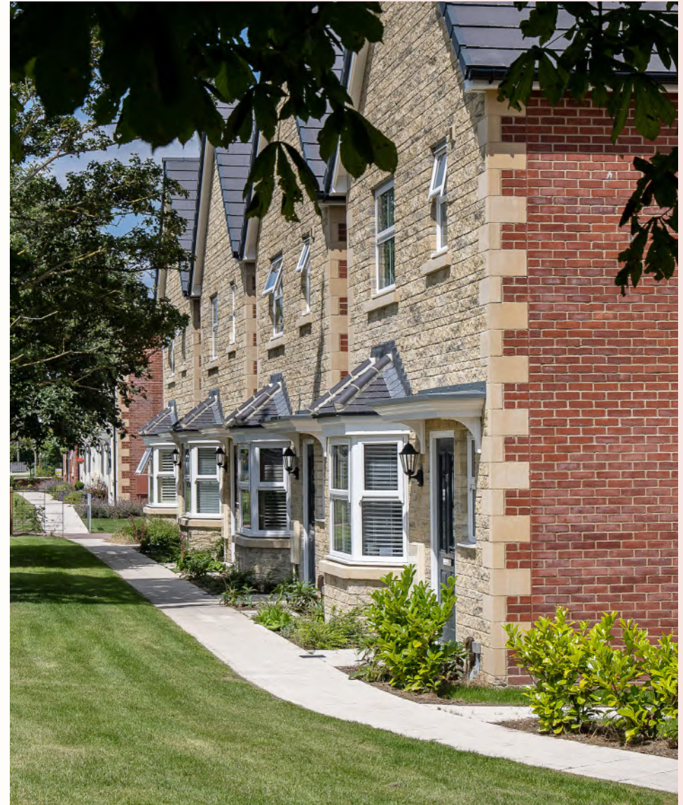
Newland Place, Trowbridge
