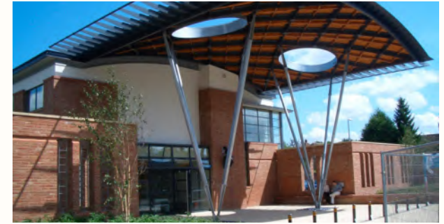
Wiltshire Police Station, Trowbridge
