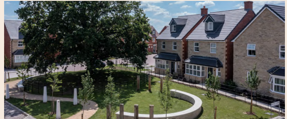
Newland Place, Trowbridge
