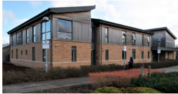
Trowbridge Health Centre
